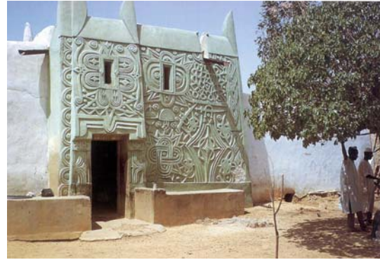
Dwellings and Settlements. Fig. 6 Decoration on the façade of a Hausa merchant's house, Zaria, Nigeria (Source: Paul Oliver, Encyclopedia of Vernacular Architecture of the World , p. 581) (Courtesy of Paul Oliver).
